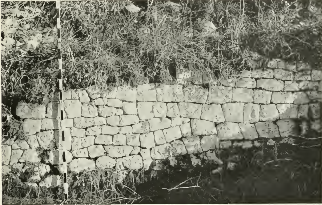
FIGURE 16. — A WALL OF OPUS INCERTUM AT 33 Now destroyed
